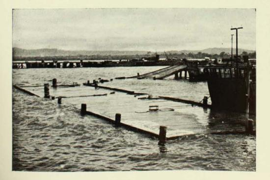
Built of unsuitable timber, this wartime Naval jetty at Ladava, New Guinea, collapsed less than 16 months after construction because of attacks on its piling by Cobra borers.
